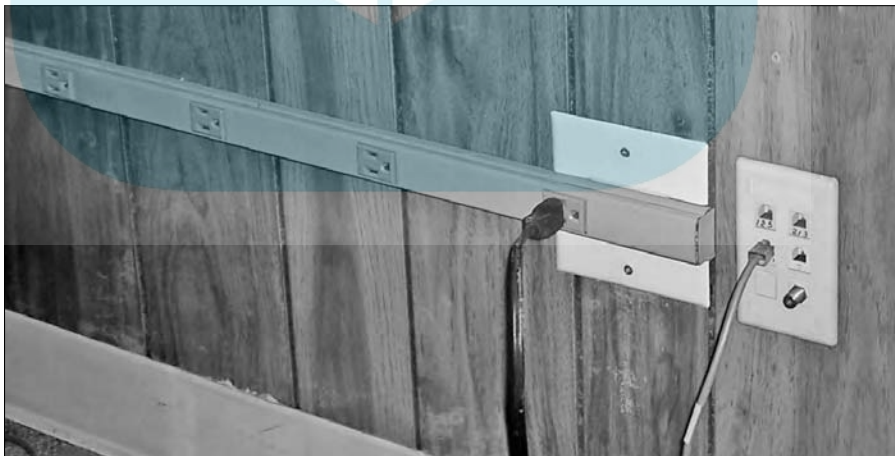
Figure 3-5: This Wiremold outlet strip can be mounted under the kitchen's upper cabinets.
